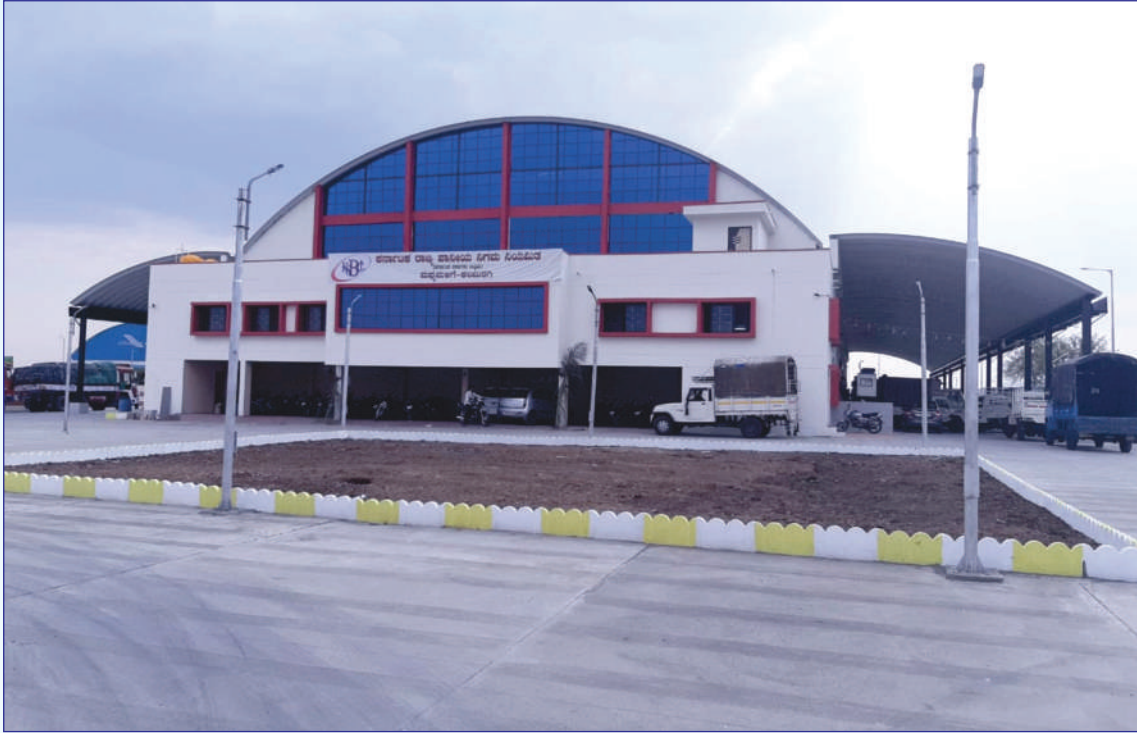
New Depot at Kalburgi
